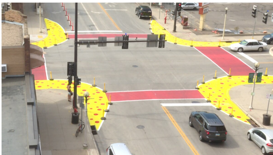
Figure 3. Image of an example of painted crosswalks and bulb-outs
