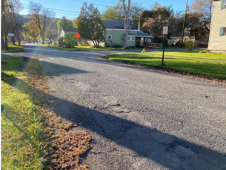
Image 9. Areas along East South Street.
