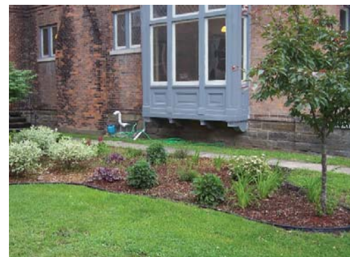
Rain garden uses runoff from the Montour Falls Library building, reducing flow into the storm sewer system.
