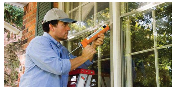
According to NYSERDA, sealing and insulating cracks in outside windows, walls, ceiling and floors can save homeowners up to 20% in heating and cooling costs. Photo Source: www.communityservices.nd.gov .
