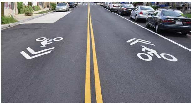
Sharrows, pictured in white paint on the road, are an affordable and effective means of letting motorists that they are sharing the road with bicycles. Sharrows can be used when the road is too narrow for designated bike lanes. Photo Source: www.mywheelsareturning.com .
