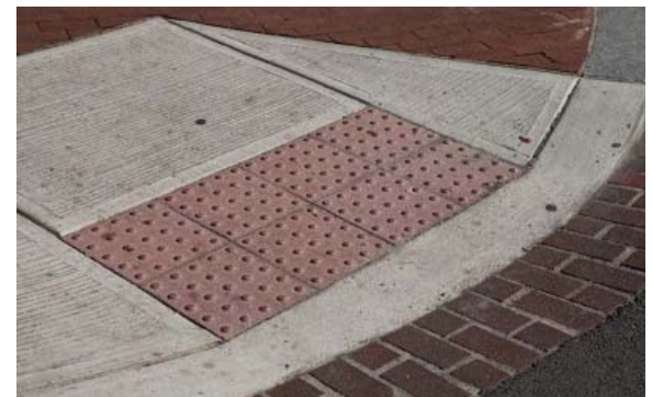
Truncated domes on a curb cut provide guidance to the visually impaired and traction to pedestrians when sidewalks are icy Photo Source: www.philly.curbed.com .
