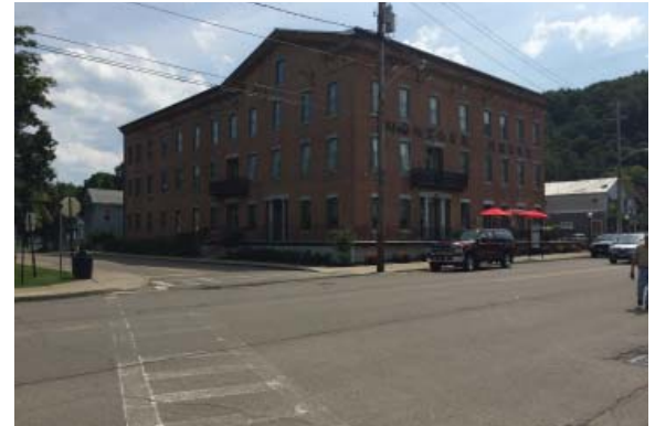
The paint has worn away at this crosswalk on Main Street, reducing its visibility. Repainting fading crosswalks is cost-effective and enhances visibility. Easily-distinguishable crosswalks alert drivers to the presence of pedestrians and make it safer for them to cross the street. Source: STC Planning Board.
