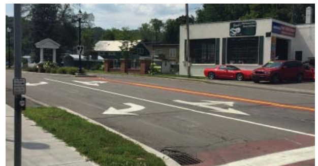
The current intersection of Main Street and Route 14. While there are elements of a complete street in place such as truncated domes, a crosswalk and sidewalks, these features do not continue for the whole length of both streets. Other elements can be added, such as street trees to slow traffic and bike lanes. Photo Source: STC Regional Planning Board.
